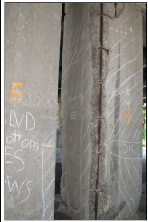
PIER 1 COLUMN 4 EAST FACE
