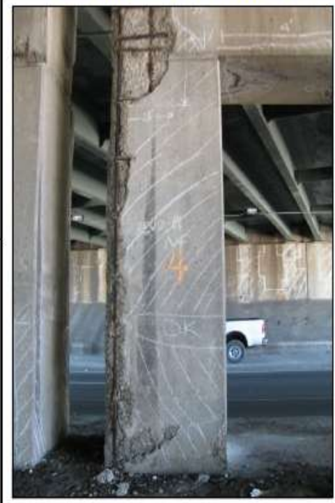
PIER 1 COLUMN 4 NORTH FACE
